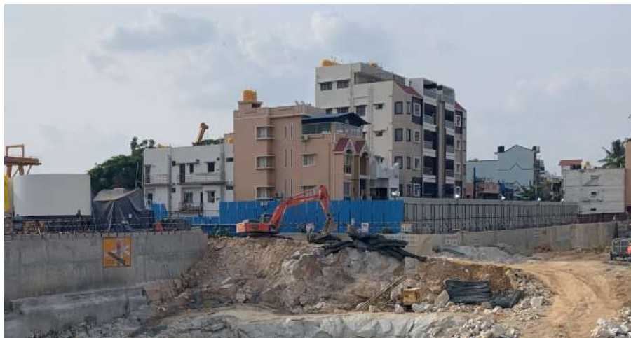
Figure 2: Some important structures around rock excavation.
