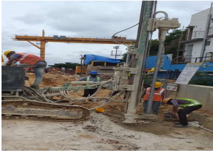
Figure 6: (Step .1). Drilling work for Presplit line.
