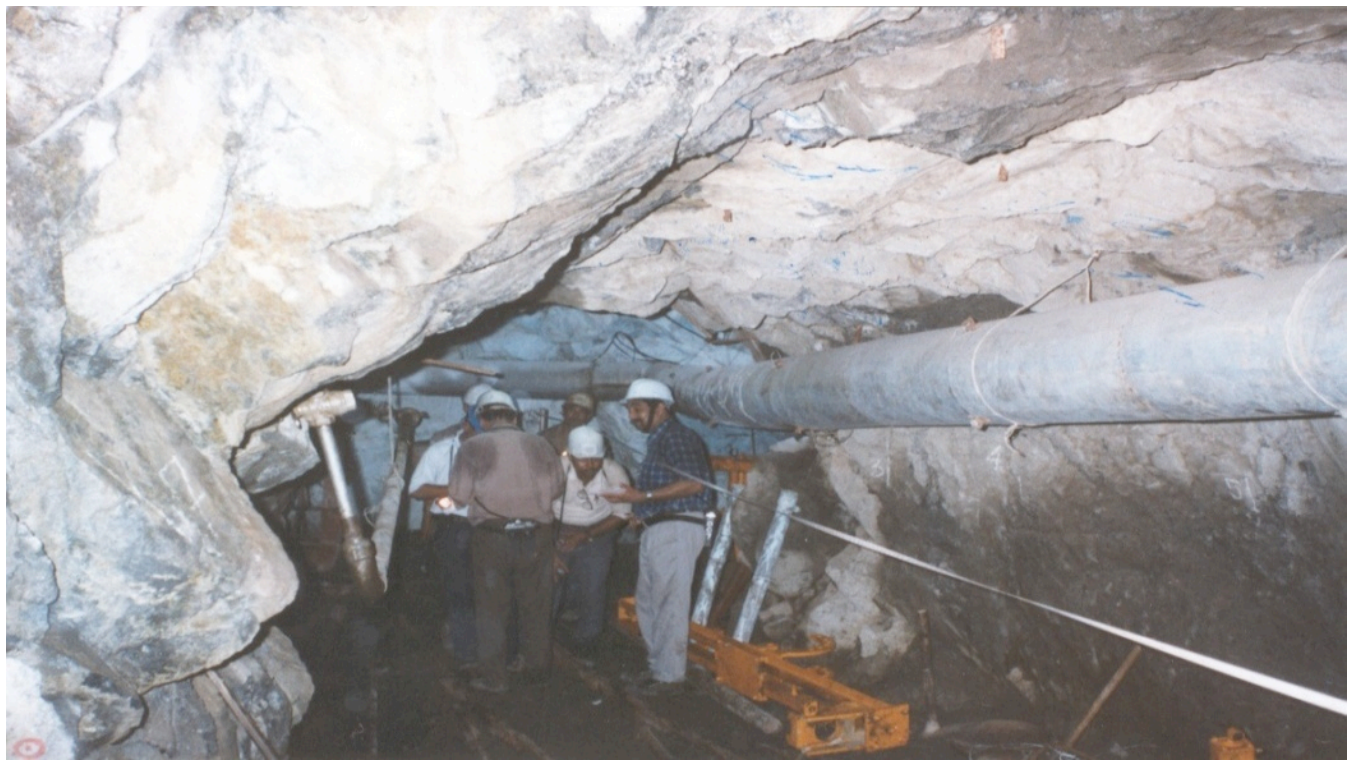
Figure 3: Scan line surveys for mapping joints in underground.
