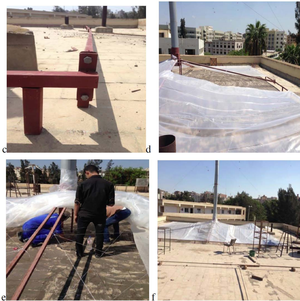
Figure 2: Pictures are showing the construction steps of the collector.
