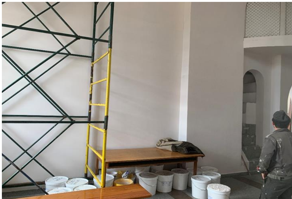
Figure 5: View after repair and painting.
