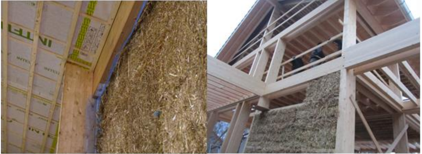
Figure 7: Showing examples of straw application of straw bale as infill wall in timber post and beam construction. Architecture barchi Belgium [Source Author].
