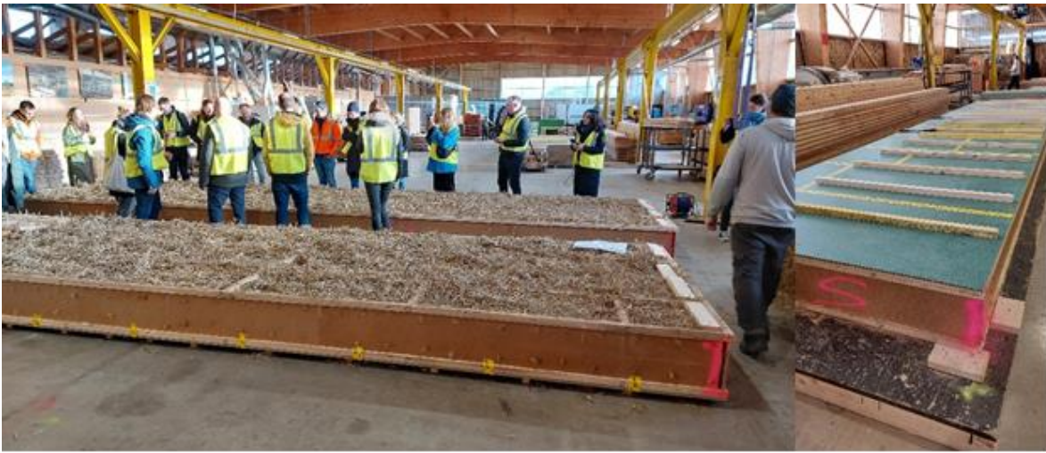
Figure 11: Showing straw bale modular wall system in manufacture with straw bale installation LHS and complete panel RHS. Chênelet northern France [Source Author].
