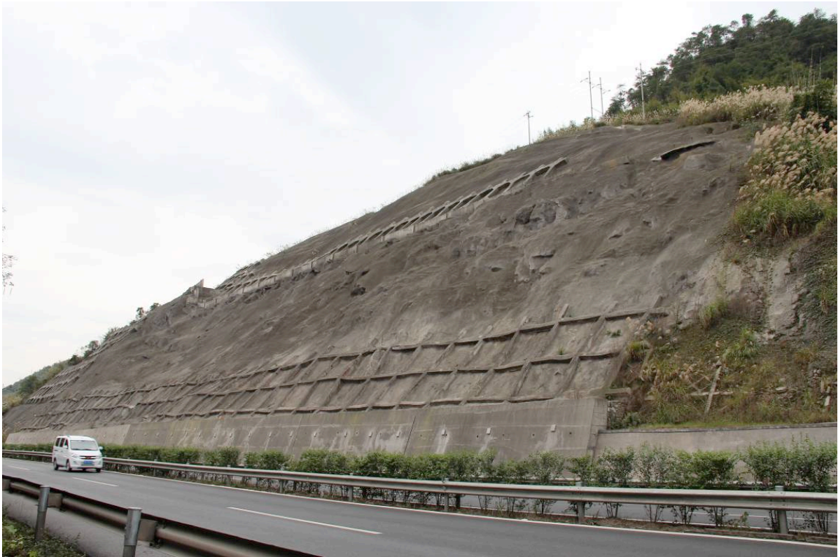
Figure 8: Photo of rock slope after near 3 years since stabilization.
