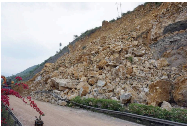
Figure 3: Photo of rock slope after failure (on May 4, 2013).
