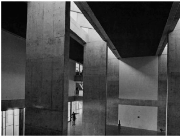
Figure 28: The original exhibition space lighting design of Le Corbusier's Museum and Art Gallery in Chandigarh. Note the absence of lights below the clerestory.
