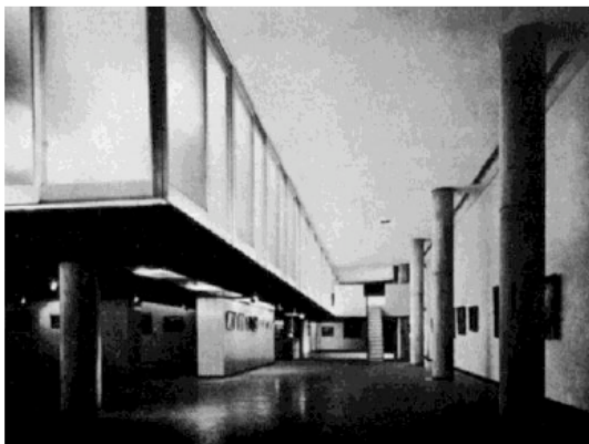
Figure 23: The original exhibition space lighting design of Le Corbusier's Tokyo Museum of Western Art. Note the absence of lamps on the ceiling.
