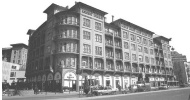
Figure 1: Architect Kemalettin Bey, Foundation Apartment, Ankara, 1926-27.
